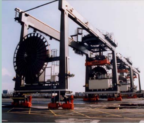
APL Pier 300 Terminal, Los Angeles
